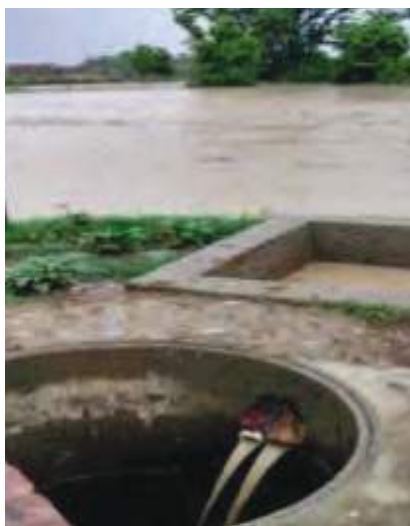
▲ Low-cost technology for dilution of groundwater through artificial recharge
