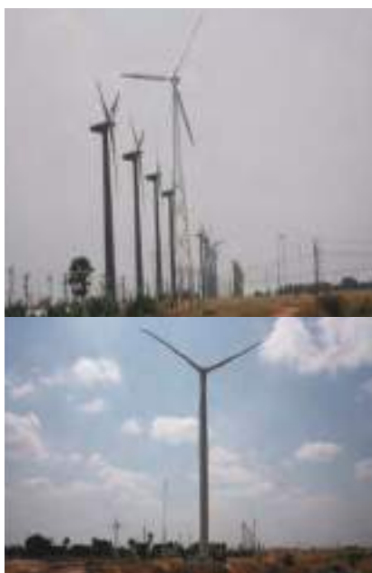
▲ 9Nos. 200kW & 1 Nos. of 600 kW constant speed 2 Nos of 2000 kW variable speed (DFIG & Syn.Gen) wind turbines
