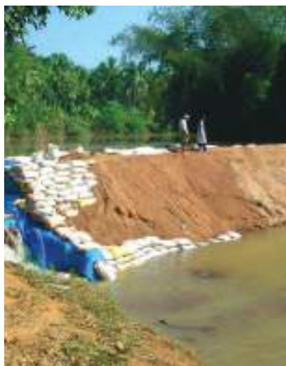
▲ Varanashi sand and plastic barrage a temporary dam designed to store water during summer months.
