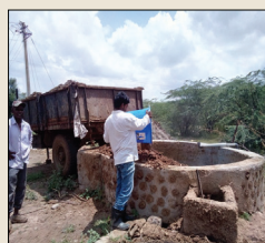
The By Product waste is dumped in the slurry tank for semi anaerobic digestion of the organic waste
