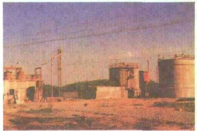
11.7 Distillery Spentwash Biomethanation pilot plant.
