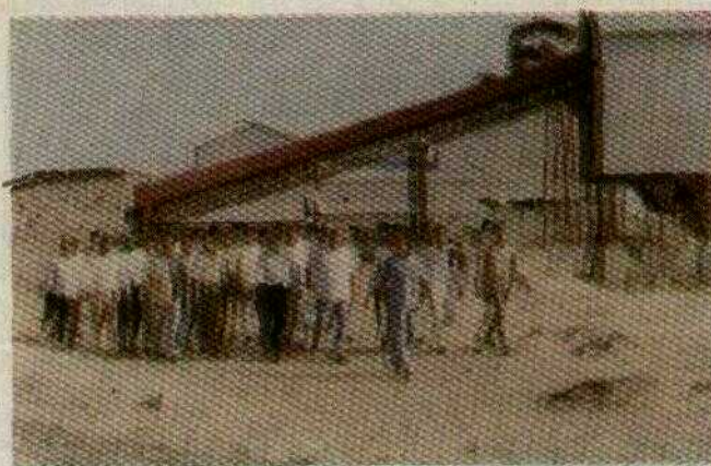
VIII.A.2 A view of the sand lime brick plant at Dungargarh (Rajasthan)
