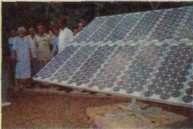
VII.B.2 SPV operated deep well pump installed by CEL in village La-Magalina, Cuba.
