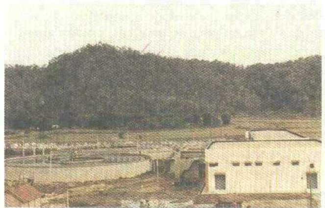
V.A. 2 Waste Water Settling Tank
