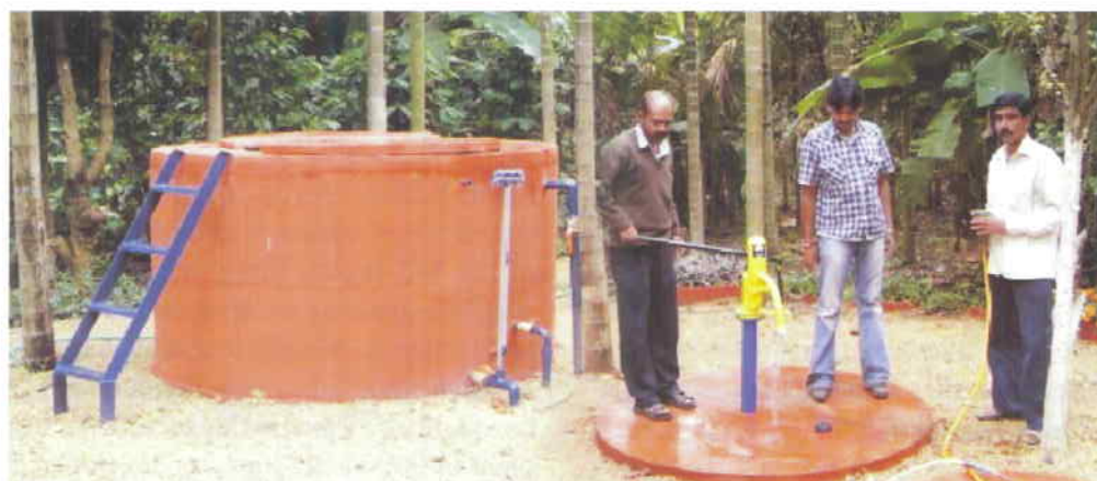
Fig. 45: Terafil Water Purification Plant with a capacity of 5000 Lt. per day installed in Karnataka
