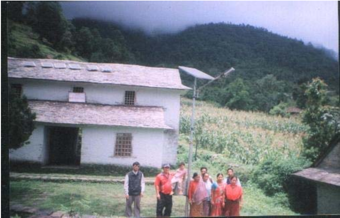
A View of the Village Jaljala (Nepal) Electrified Through Solar Energy
