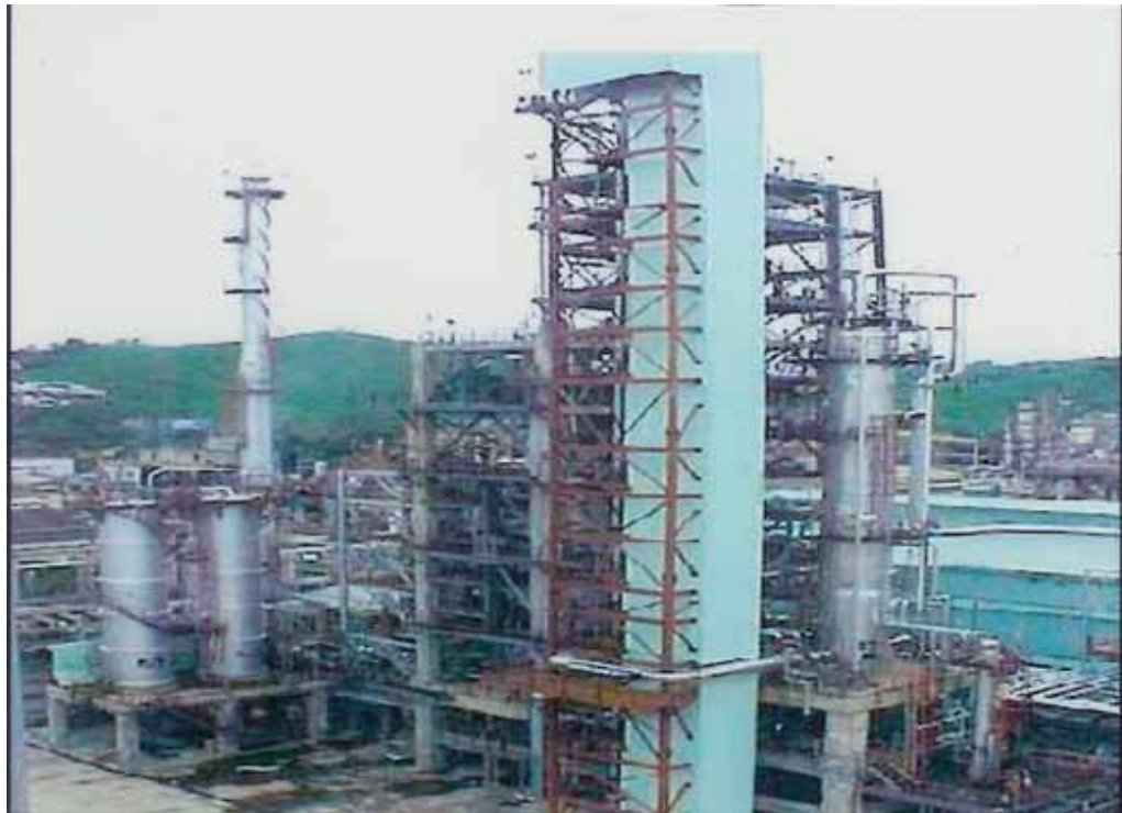
INDMAX Unit at Guwahati Refinery
