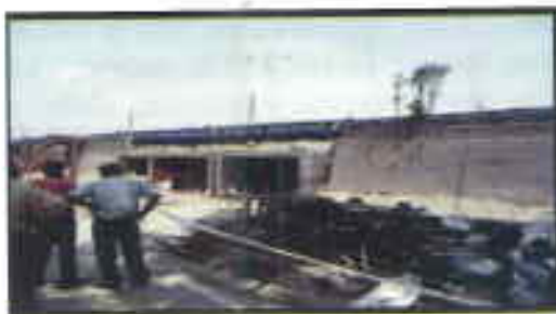
Train Movement on Completed Underpass
