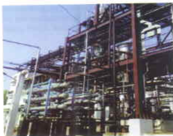
Fig. 1.24. Based on the process developed by CSIR-NEERI, a full scale ETP of 600 m 3 /d design capacity comprising (A) ammonia stripper and (B) Two Stage Biooxidation (TSB) process has been implemented at Nagarjuna Agrichem Ltd, Srikakulam
