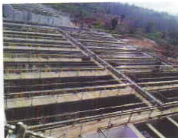
Fig. 1.24. Based on the process developed by CSIR-NEERI, a full scale ETP of 600 m 3 /d design capacity comprising (A) ammonia stripper and (B) Two Stage Biooxidation (TSB) process has been implemented at Nagarjuna Agrichem Ltd, Srikakulam
