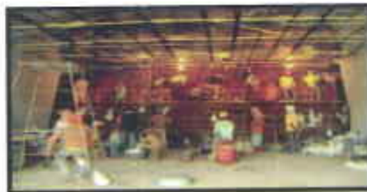
Inside View of the Box during Pushing
