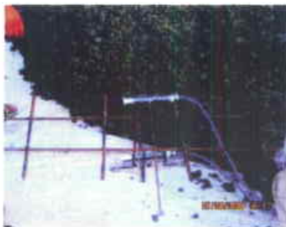
Sensors Embedded in Concrete Pavement
