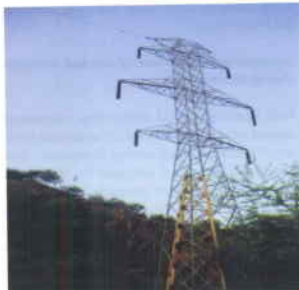
Fig. 1.46a. Experimental Tower erected at Test Bed
