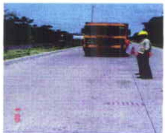
Load Testing of Instrumented Pavement
