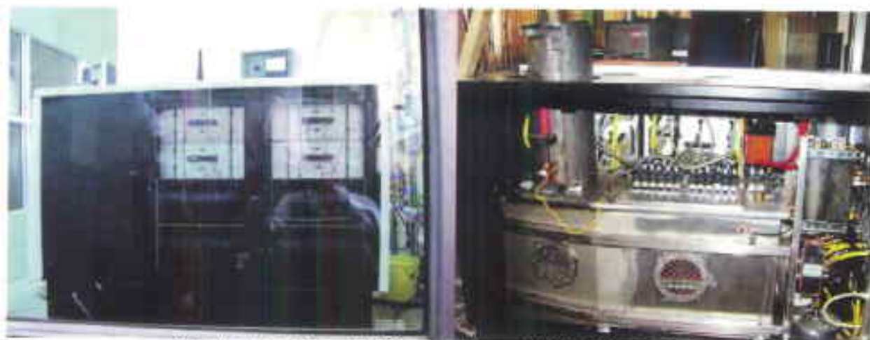
Fig. 1.83. High Voltage Solid State Modulator with GCTM Under Testing
