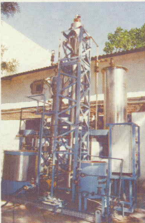
III.A.3 Pilot Plant for Fluidised Heat Exchanger
